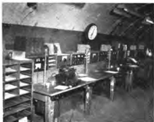
— The interior of a westward ACS station after some of the refinements of a permanent station have been installed. The ruggedness of early operation immediately after an Aleutian landing is gone. The neat filing cabinet at left, the clean-cut operating positions, the big wall clock and the fluorescent lighting — all are a far cry from the mud-floored tent in use when this station was first established.
